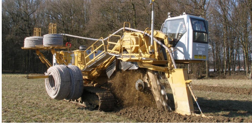
Figure 2.9 Chain trencher machine installing prewrapped geotextile (PLM) drainpipe (Mastenbroek, 2022).
