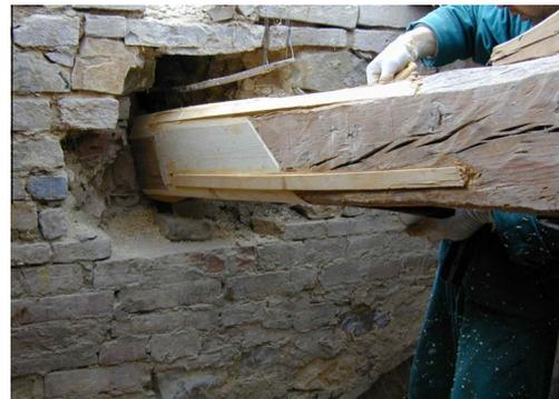
**Fig. 5.** Insertion of a final wedge.
