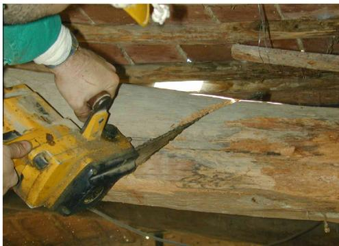
**Fig. 3.** Inclined cut of decayed end.
