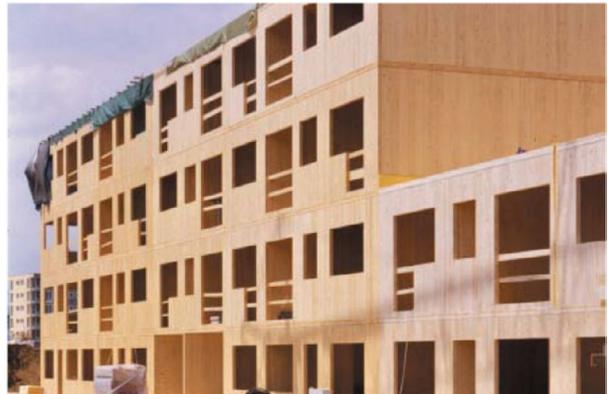
Figure 2. Manufacture, transportation and erection of CLT panels [Images: KLH].
