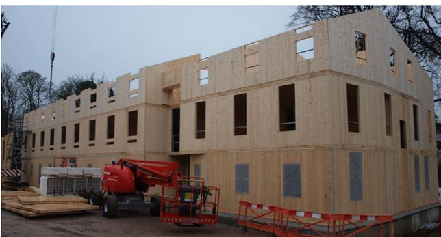
Figure 3. Platform construction [Image: C UíChúláin].
