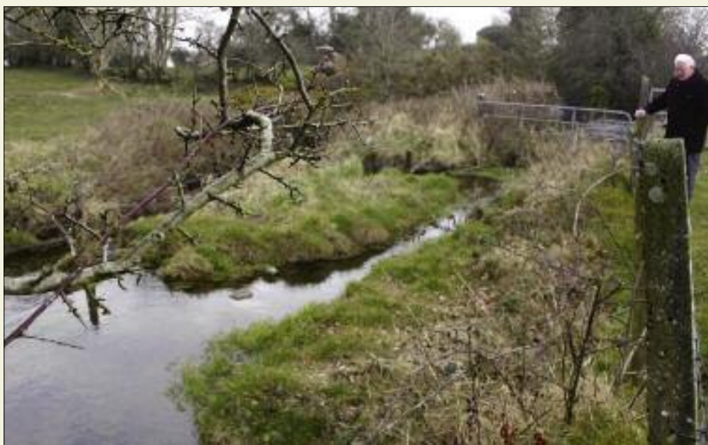
Above: Michael John Kilgannon at the abstraction point from the river that would serve as a source for 40 years. Opposite page: The old pump house on a site donated by the landowner to the scheme free-of-charge.
