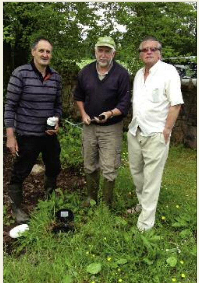
Meter installation on Ballinguyroe & Tankardstown GWS.
