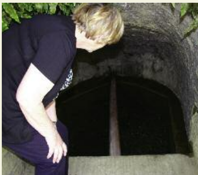
Phyllis Naughton of Ballinamona GWS at a former groundwater source of drinking water for the scheme that was abandoned due to contamination.
