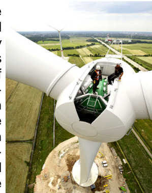
Hub of a 5 MWatt Wind Turbine
