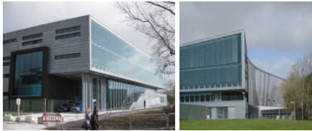
Figure 1: The recently completed New Engineering Building at the National University of Ireland, Galway
